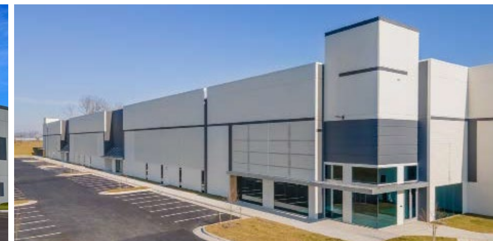
Parkway 66 High Bay Warehouse, Manassas, VA
