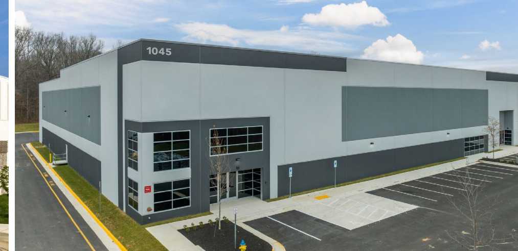
Crossroads Industrial High Bay Warehouse, Fredericksburg, VA
