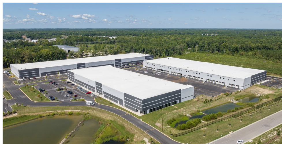
Northlake II 5-Building, 655,000 SF Industrial Park
