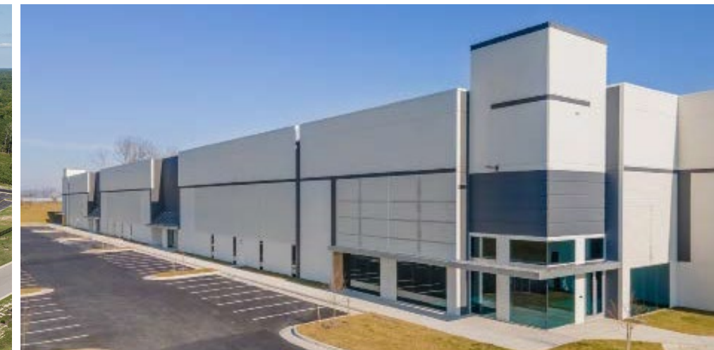
Parkway 66 High Bay Warehouse, Manassas, VA
