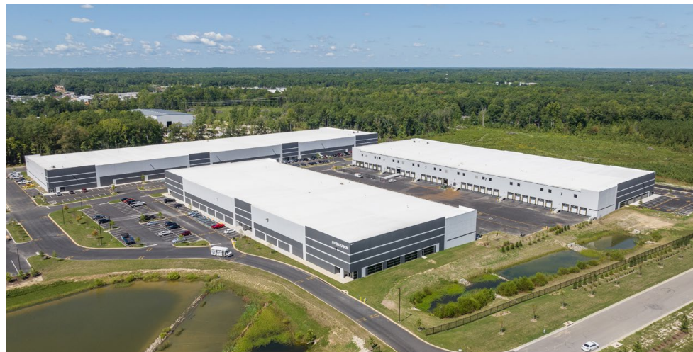
Northlake II 5-Building, 655,000 SF Industrial Park
