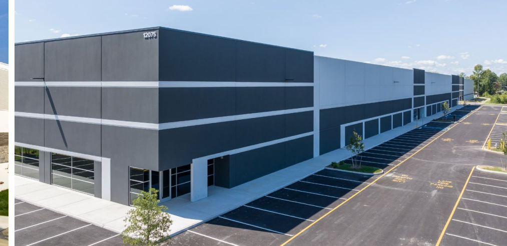
Northlake II 5-Building, 655,000 SF Industrial Park
