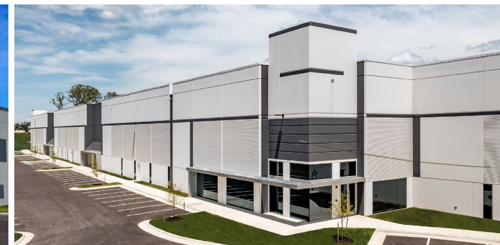
Parkway 66 High Bay Warehouse, Manassas, VA
