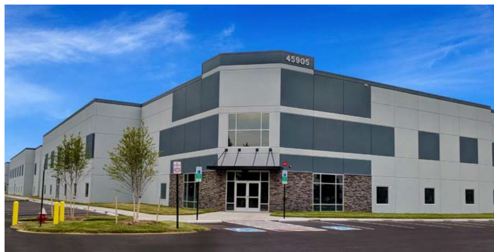
Dulles North High Bay Warehouse, Sterling, VA
