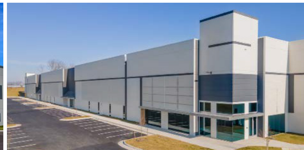
Parkway 66 High Bay Warehouse, Manassas, VA
