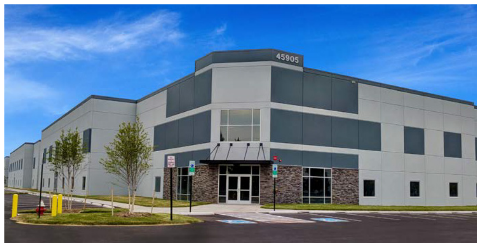
Dulles North High Bay Warehouse, Sterling, VA
