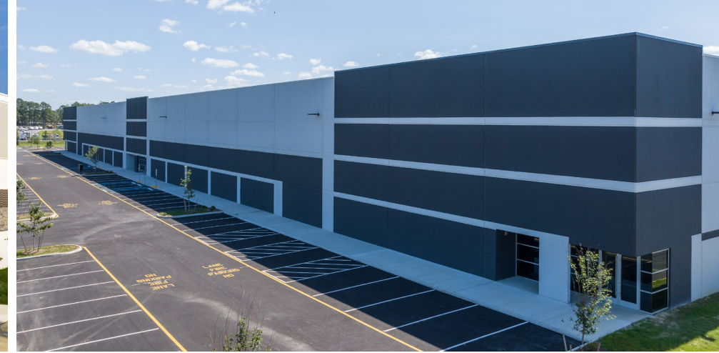
Northlake II 5-Building, 655,000 SF Industrial Park
