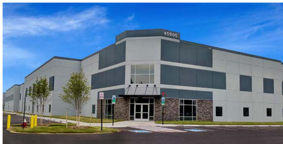
Dulles North High Bay Warehouse, Sterling, VA
