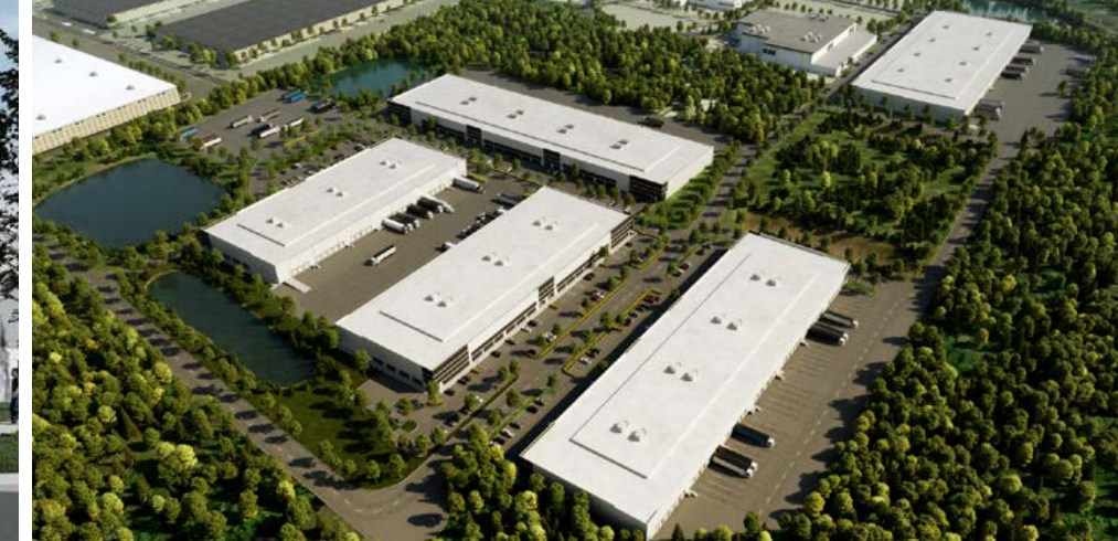
Northlake II 5-Building, 655,000 SF Industrial Park
