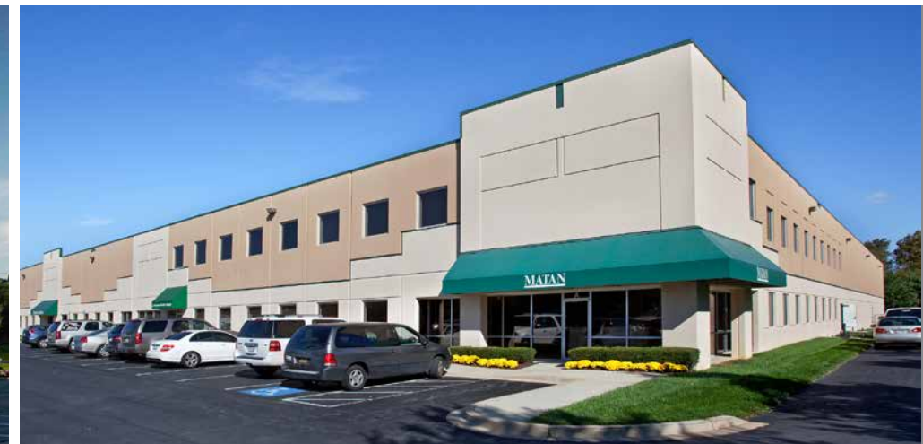
Matan Headquarters Wedgewood II
