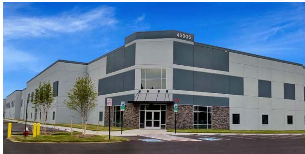
Dulles North High Bay Warehouse, Sterling, VA
