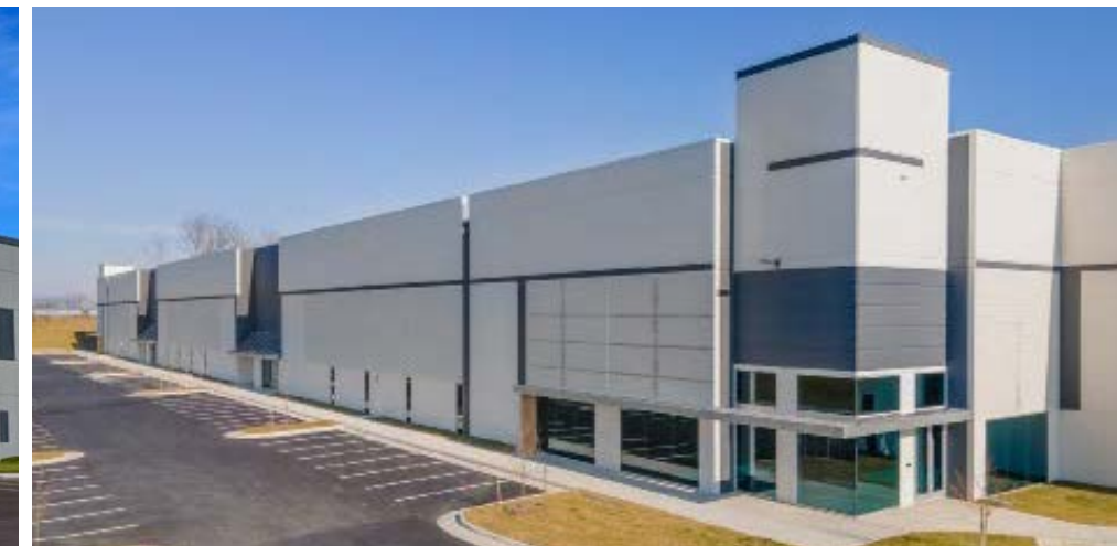
Parkway 66 High Bay Warehouse, Manassas, VA
