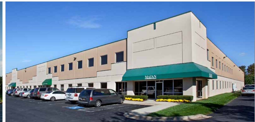
Matan Headquarters Wedgewood II
