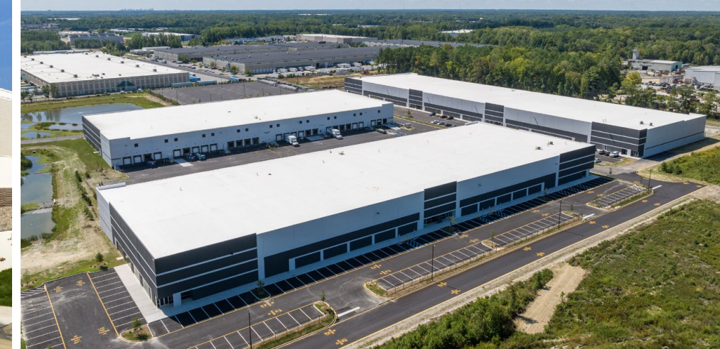
Northlake II 5-Building, 655,000 SF Industrial Park
