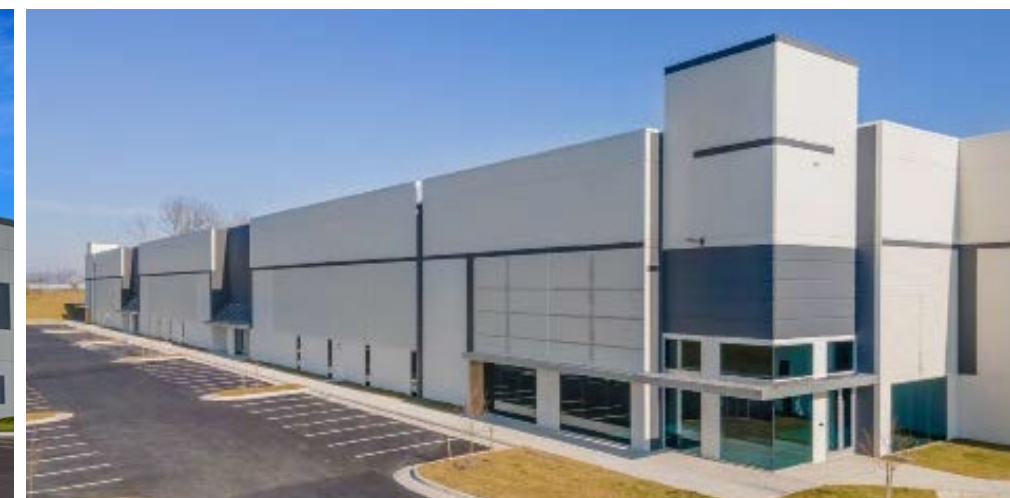
Parkway 66 High Bay Warehouse, Manassas, VA
