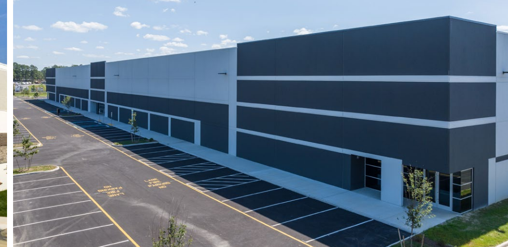
Northlake II 5-Building, 655,000 SF Industrial Park
