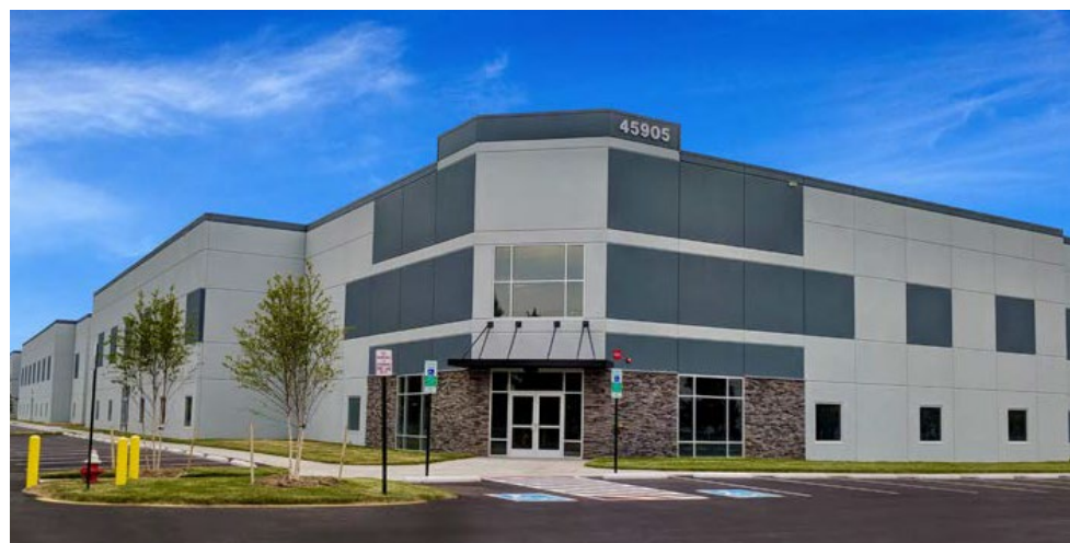
Dulles North High Bay Warehouse, Sterling, VA
