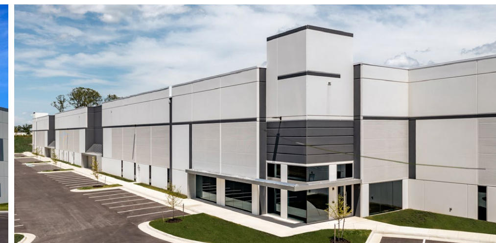
Parkway 66 High Bay Warehouse, Manassas, VA
