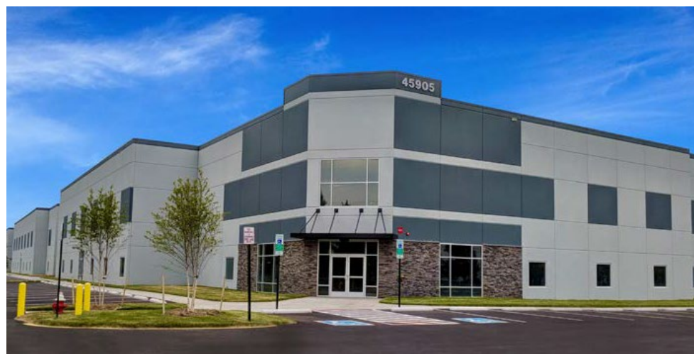
Dulles North High Bay Warehouse, Sterling, VA
