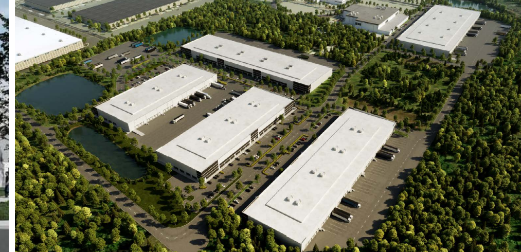
Northlake II 5-Building, 655,000 SF Industrial Park
