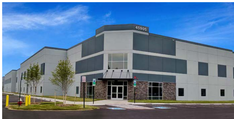
Dulles North High Bay Warehouse, Sterling, VA
