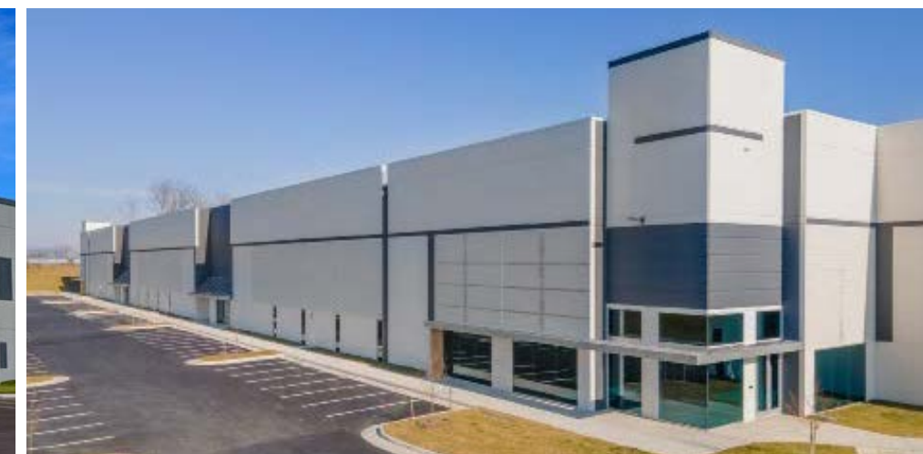
Parkway 66 High Bay Warehouse, Manassas, VA
