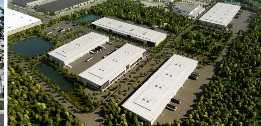
Northlake II 5-Building, 655,000 SF Industrial Park
