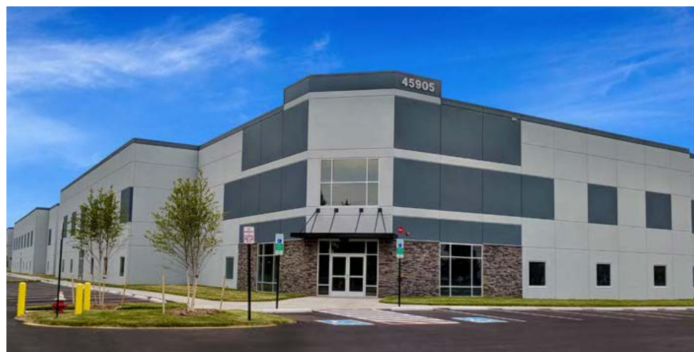
Dulles North High Bay Warehouse, Sterling, VA
