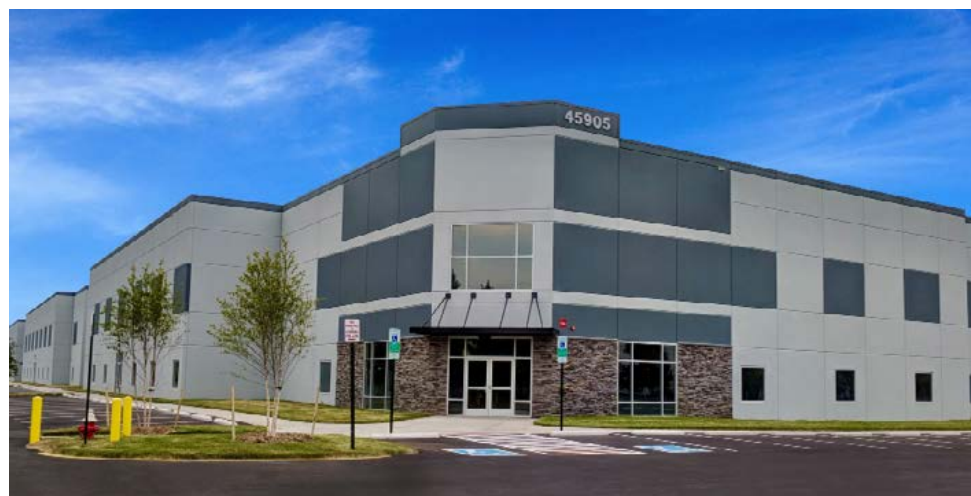
Dulles North High Bay Warehouse, Sterling, VA
